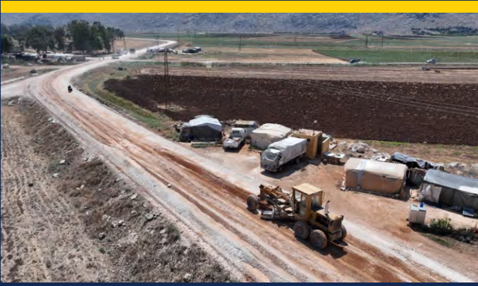
Rehabilitation of the 6-kilometer-long road from Namra intersection to Bal'a.
