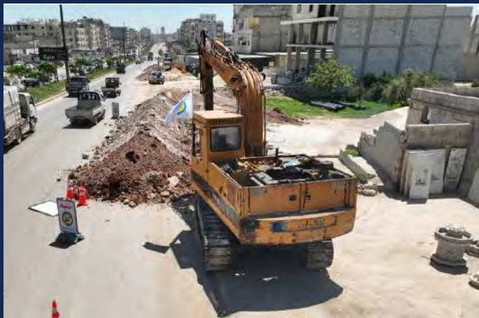
Rehabilitation of Wastewater Networks in Azaz City
