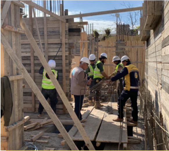
Construction of the Khalid bin Al-Walid School in Jandairis.
