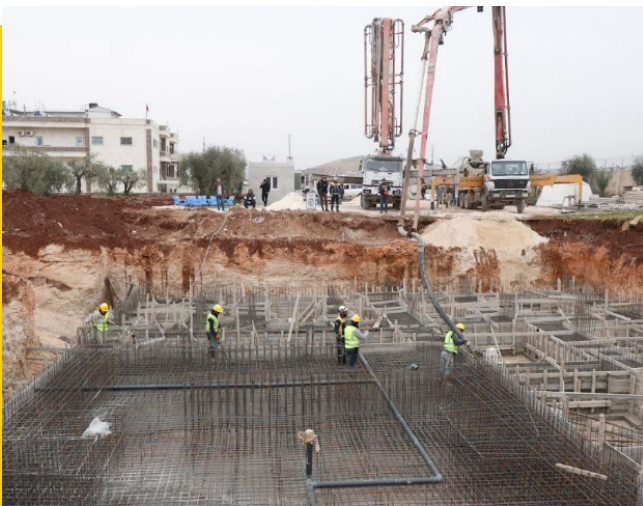
Excavation the foundations of the cancer center in Afrin.
