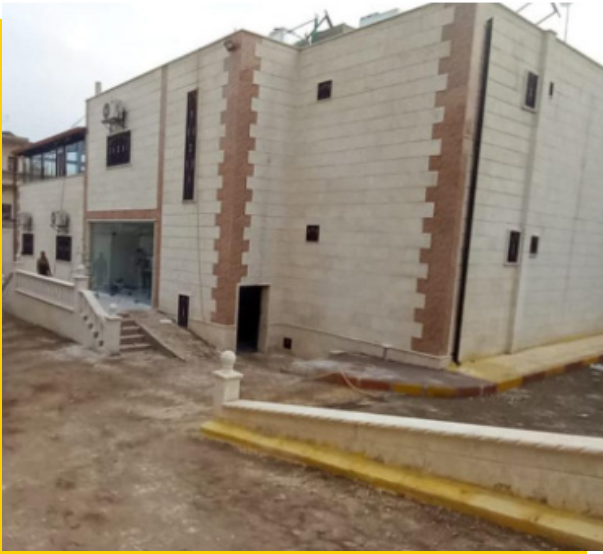
Rehabilitation of a community center in Afrin.
