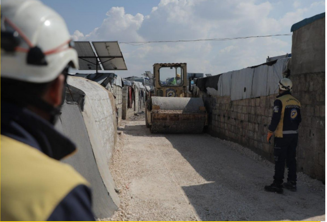
Winter response work, including land leveling and graveling in more than 50 camps affected by floods.
