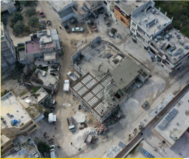
External and internal cladding work on the Al-Maland Mosque.
