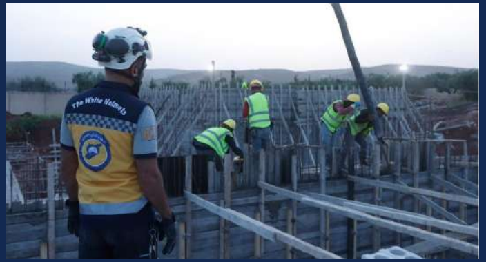
Construction of a cancer treatment center in Afrin city.
