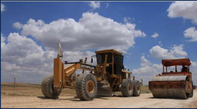
Rehabilitation of the 8.5-kilometer-long Ain al-Beida-Qandaria road.
