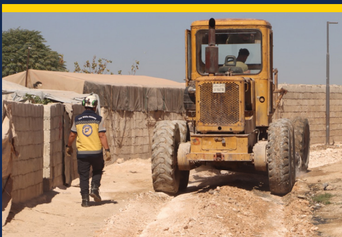
Paving and leveling roads in 25 camps.
