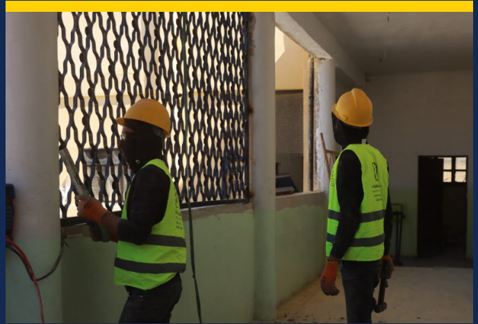
Rehabilitation of 22 Schools.
