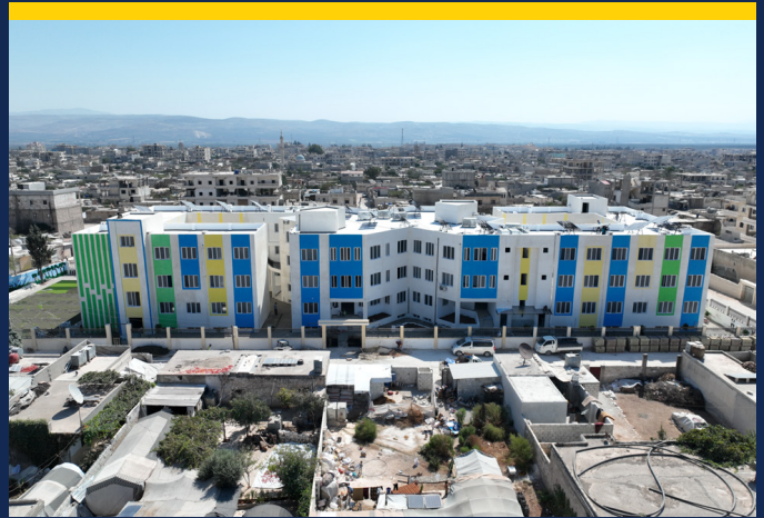
Construction of the Khalid bin Al-Walid School in Jandairis.
