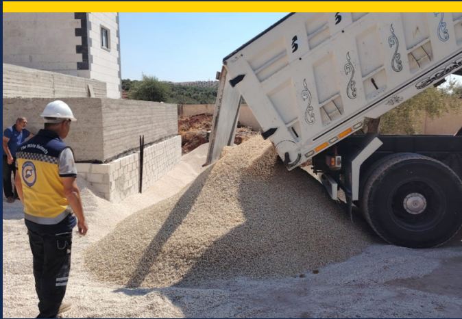
Construction of the Cancer Treatment Center in Afrin City.
