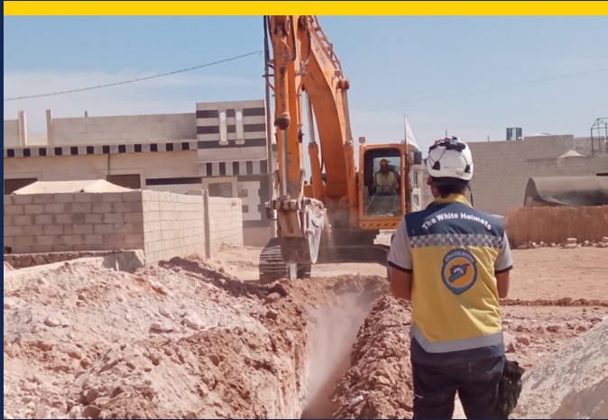
Rehabilitation of 5,050 meters of sewage networks in Al-Bab City.
