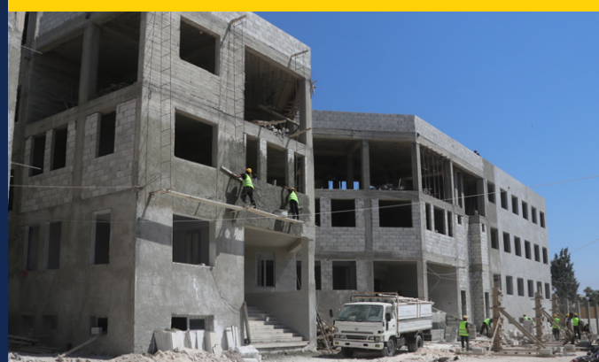
Construction of the Khalid bin Al-Walid School in Jandairis.
