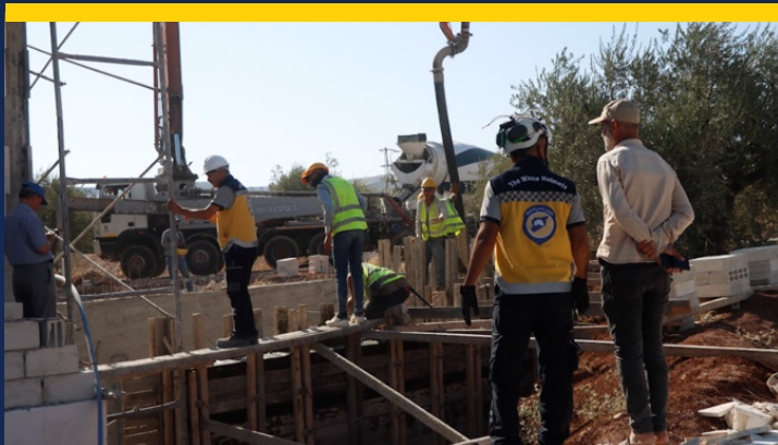
Construction of the Cancer Treatment Center in Afrin City
