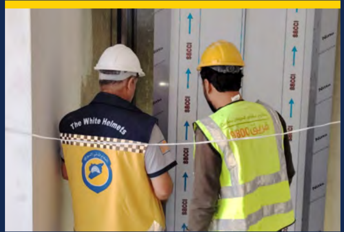
Construction of the Cancer Treatment Center in Afrin City.
