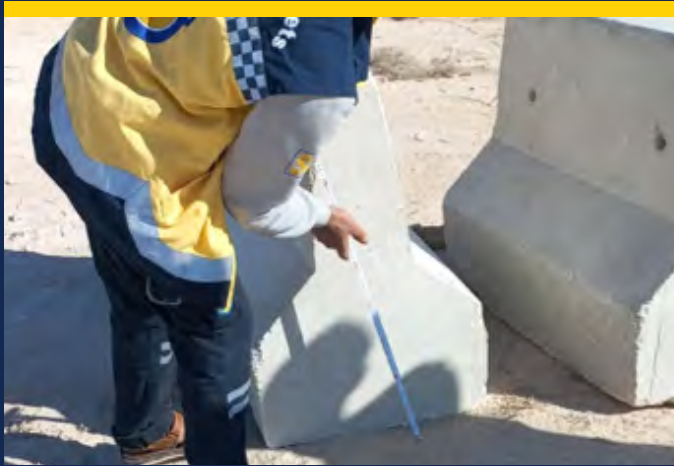
Rehabilitation of the 8.5-kilometer-long Ain al-Beida-Qandaria road.
