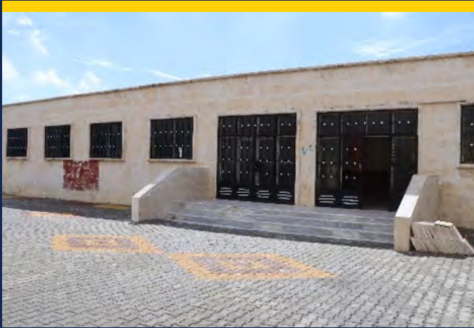
Rehabilitation of 22 earthquake-damaged schools.
