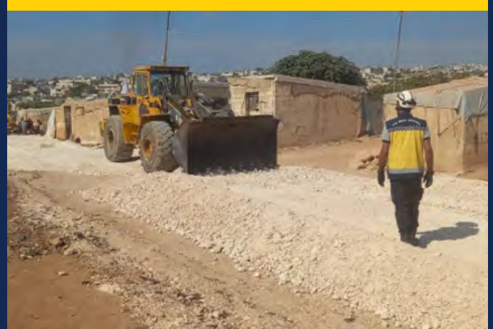
Roads rehabilitation inside camps through graveling and leveling within 25 camps
